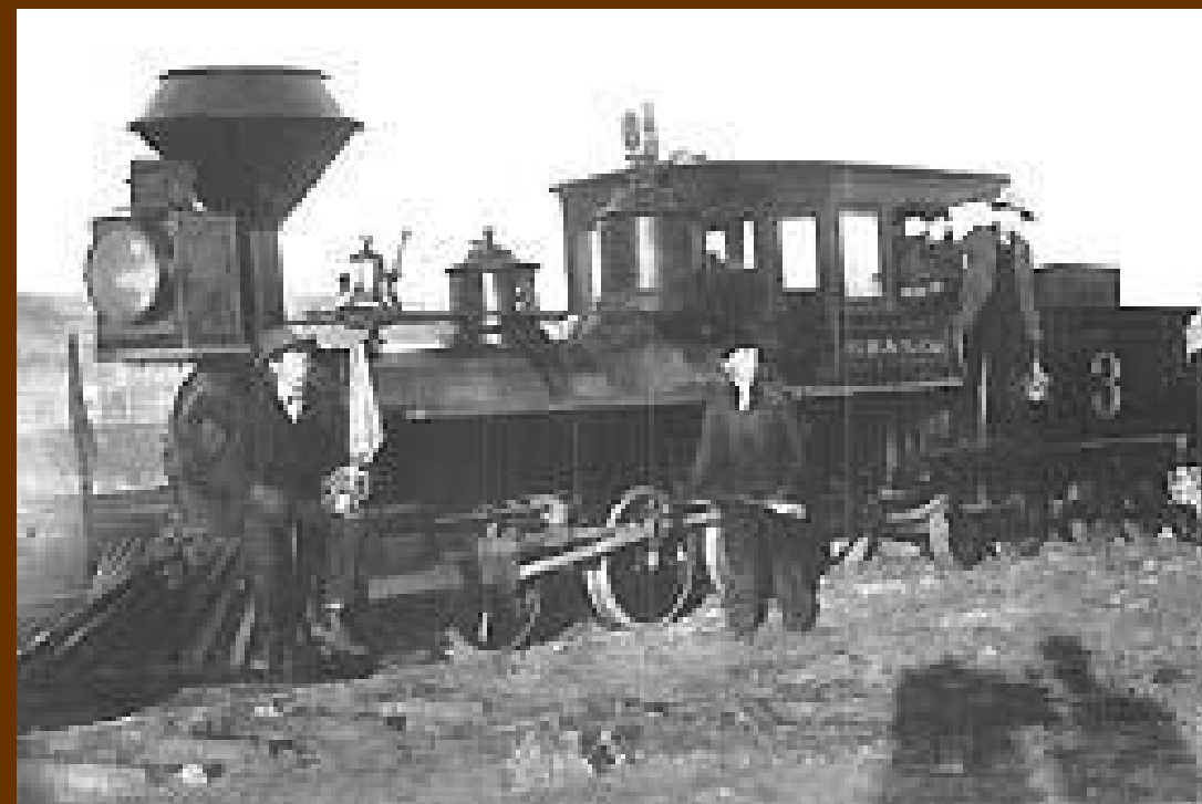
Blue Mountain engine on the Blue Mt. Extension and Mill Creek line
