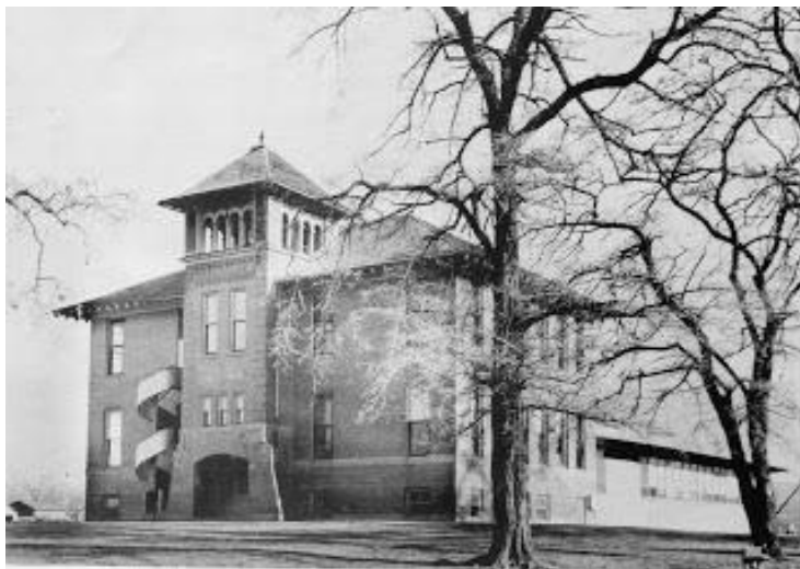
The 1910 building with 1950 addition
