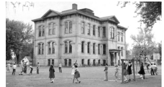
1931 remodel, photo from 1955
